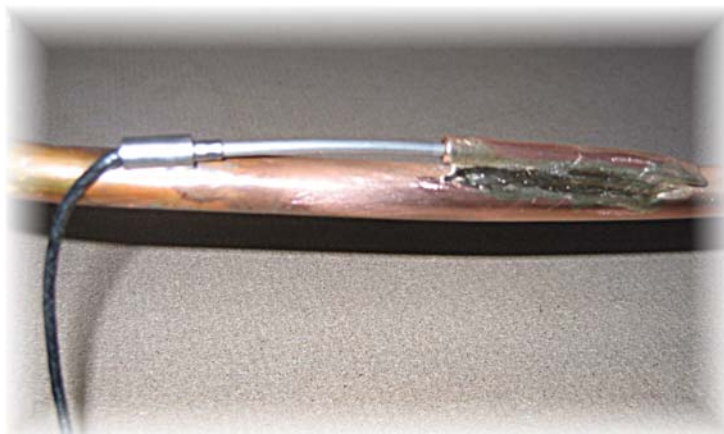
Diagram 16. Remote sensor silver soldered to refrigeration line.
